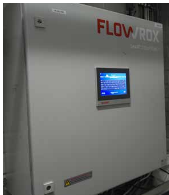
Automation system control unit, part of Malibu™ monitoring and automation system.
